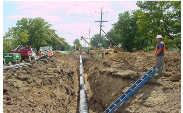
A multi-team approach was used to expedite field assessments along the entire 70-mile long corridor in a shortened timeframe.
